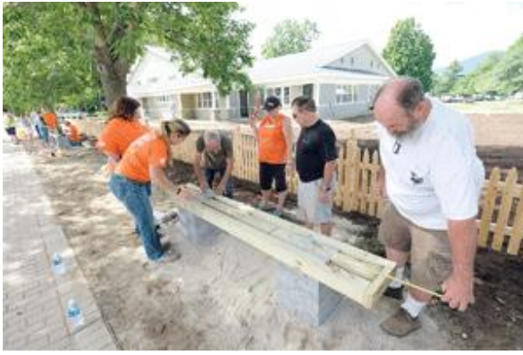
Home eot associates and eterans construct one o ie benches at the community center. (JAMIE GEMMITI PHOTO)
